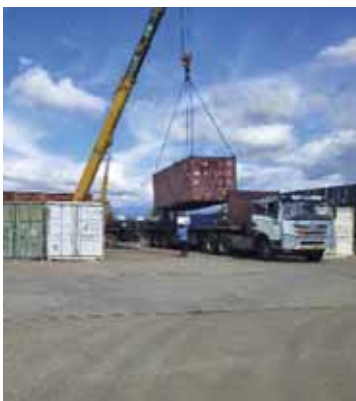
Post Ex reconditioning.
