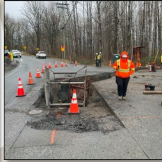
SRRMC's Kelsey Raab conducting monitoring for Schweyey Road Force Main Project.
