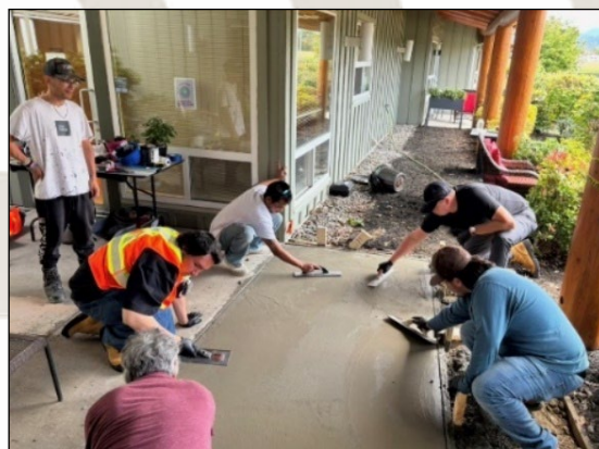
Paving completed by SASET training group.
