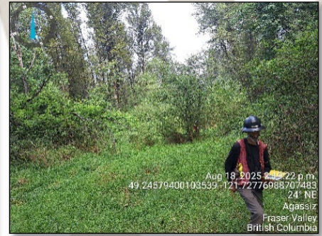
Transmountain Reclamation work.
