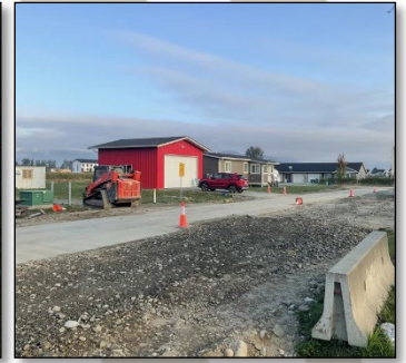
Conducting monitoring in preparation for utility installation at Yakweakwoose.
