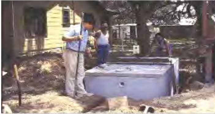
Many times an aged or failing septic system requires tank replacement (Source: Texas A&M University, 1995)
