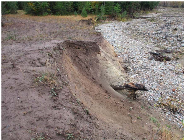
Figure 2: Cut bank where tailings erode into Lightning Creek (IDEQ, 2016).
