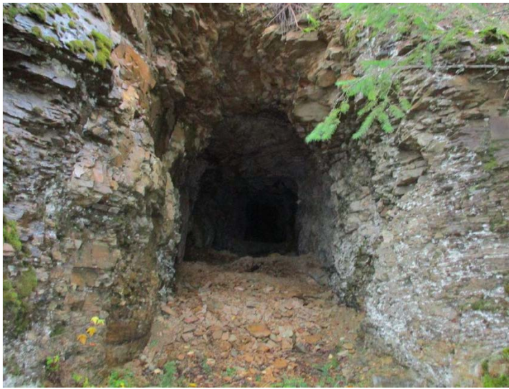
Figure 3: Photograph of Adit #1 opening (IDEQ, 2016)
