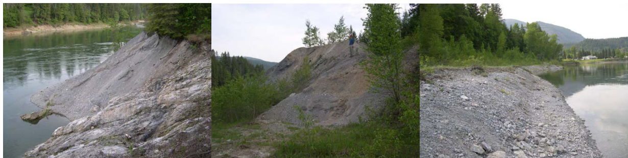
Figure 2a (left): Photograph of Waste Rock Pile #1 facing south.
