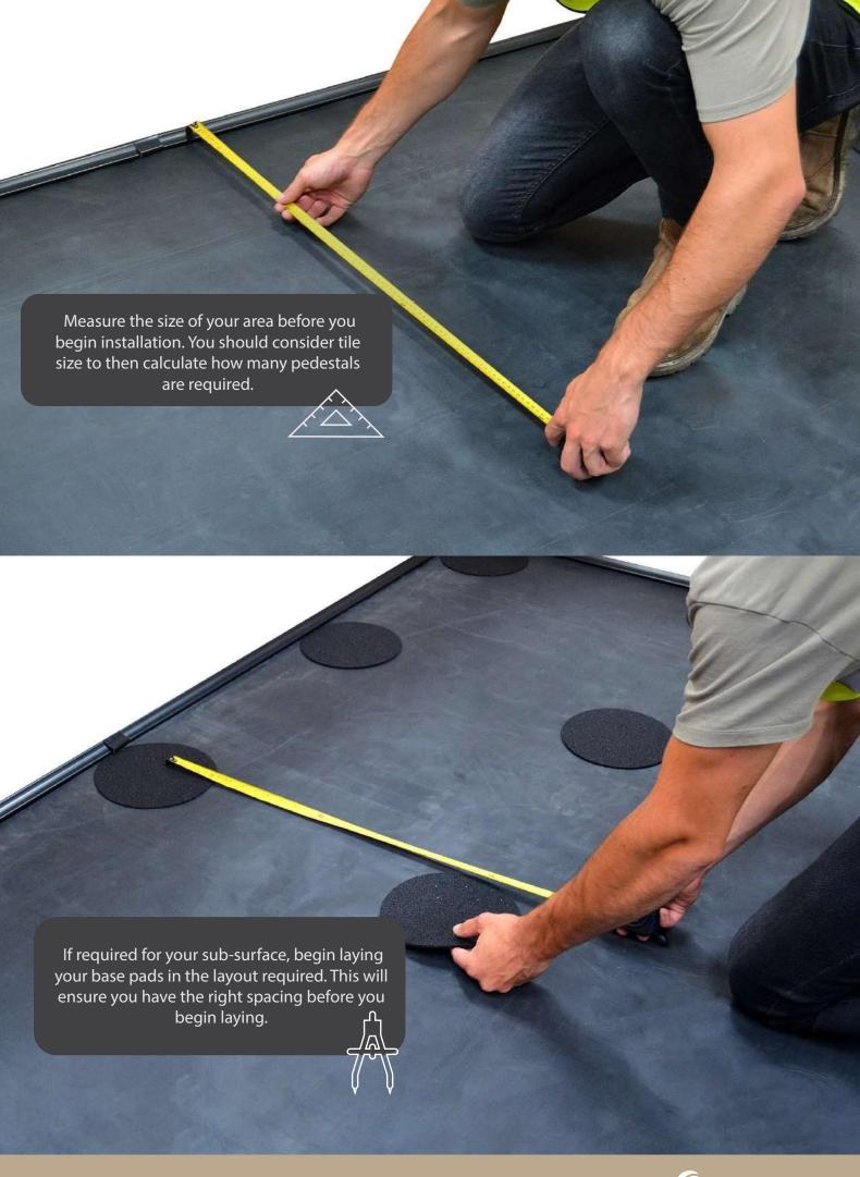
Start laying the base pads from the corner and sides of your area. You will need to remove the support tabs away from the main unit safely, using a sharp blade:
