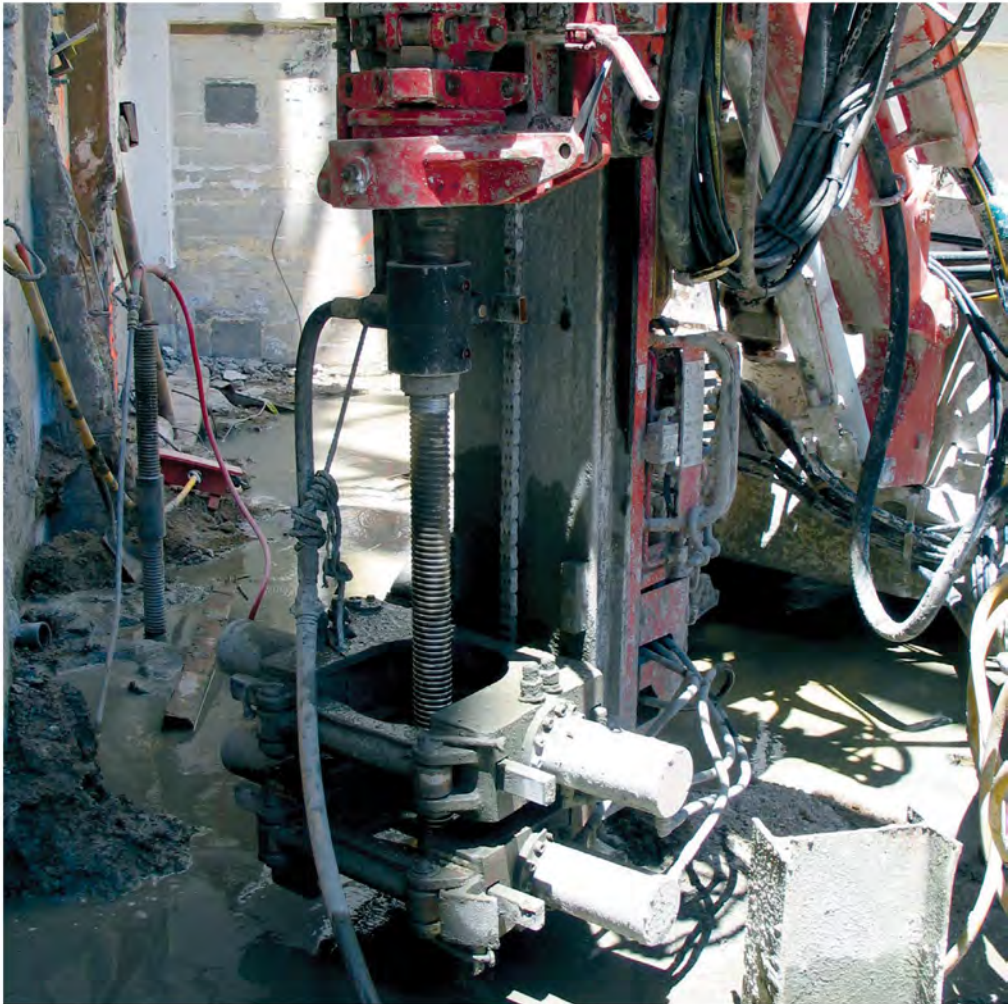
Simultaneous Drilling and Grouting
