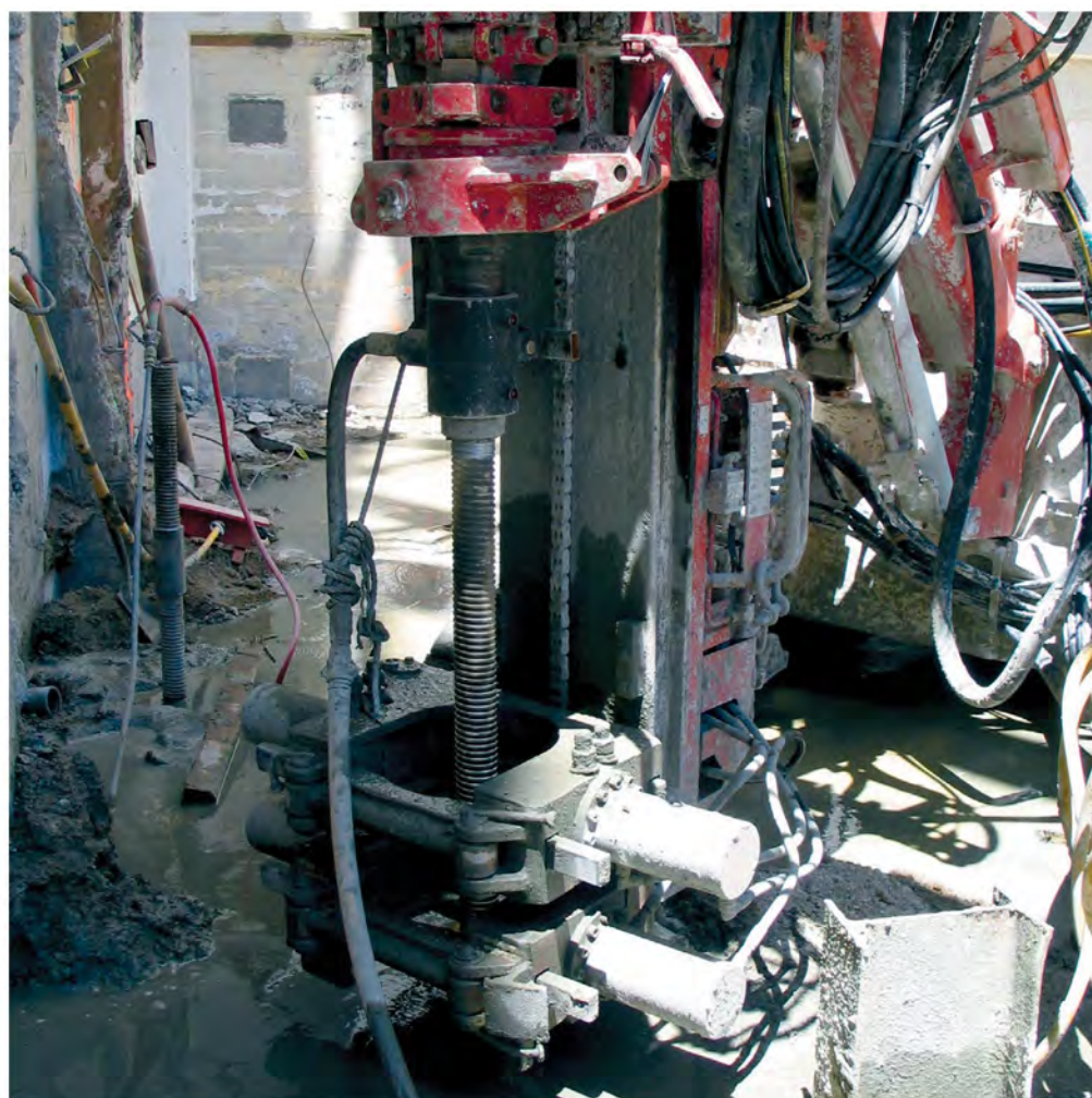
Simultaneous Drilling and Grouting
