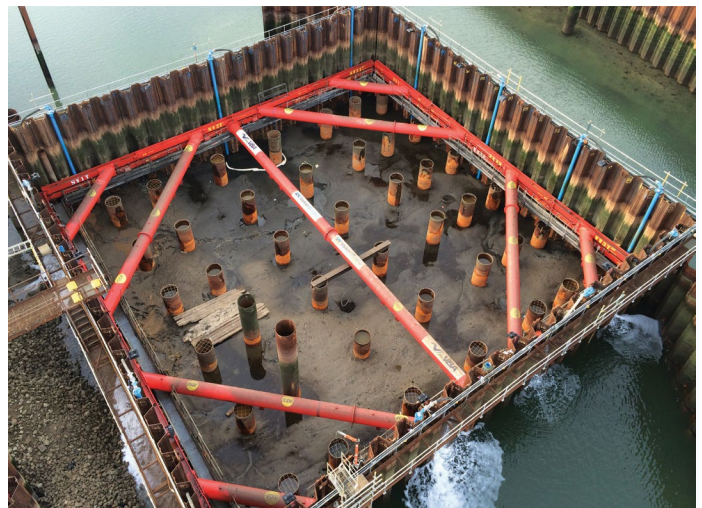
Photo: Ipswich tidal barrier, UK | ©MGF
