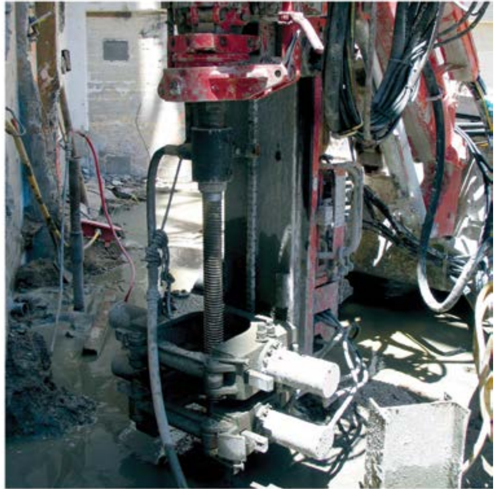
Simultaneous Drilling and Grouting
