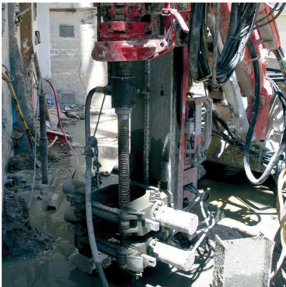
Simultaneous Drilling and Grouting
