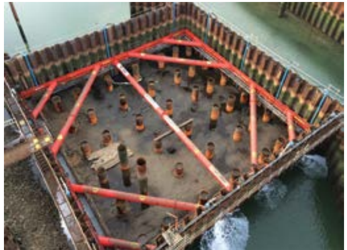
Photo: Ipswich tidal barrier, UK | ©MGF
