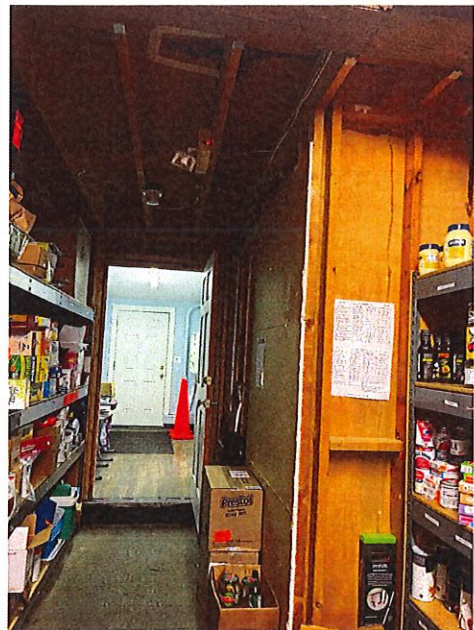
Interior Finish – Storage (note floor level)
