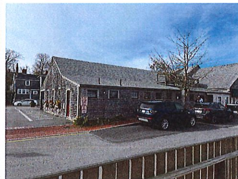
Exterior Façade – facing Candle Street
