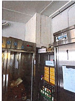
Electric Water Heater (inaccessible)
