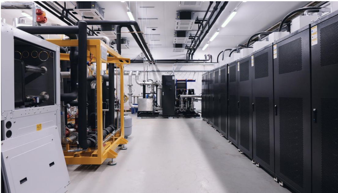
Photo at district heating facility in Satakunta, with MARA's Bitcoin mining racks enclosed on the right and heat pump equipment in the center and left. Image provided by MARA.
