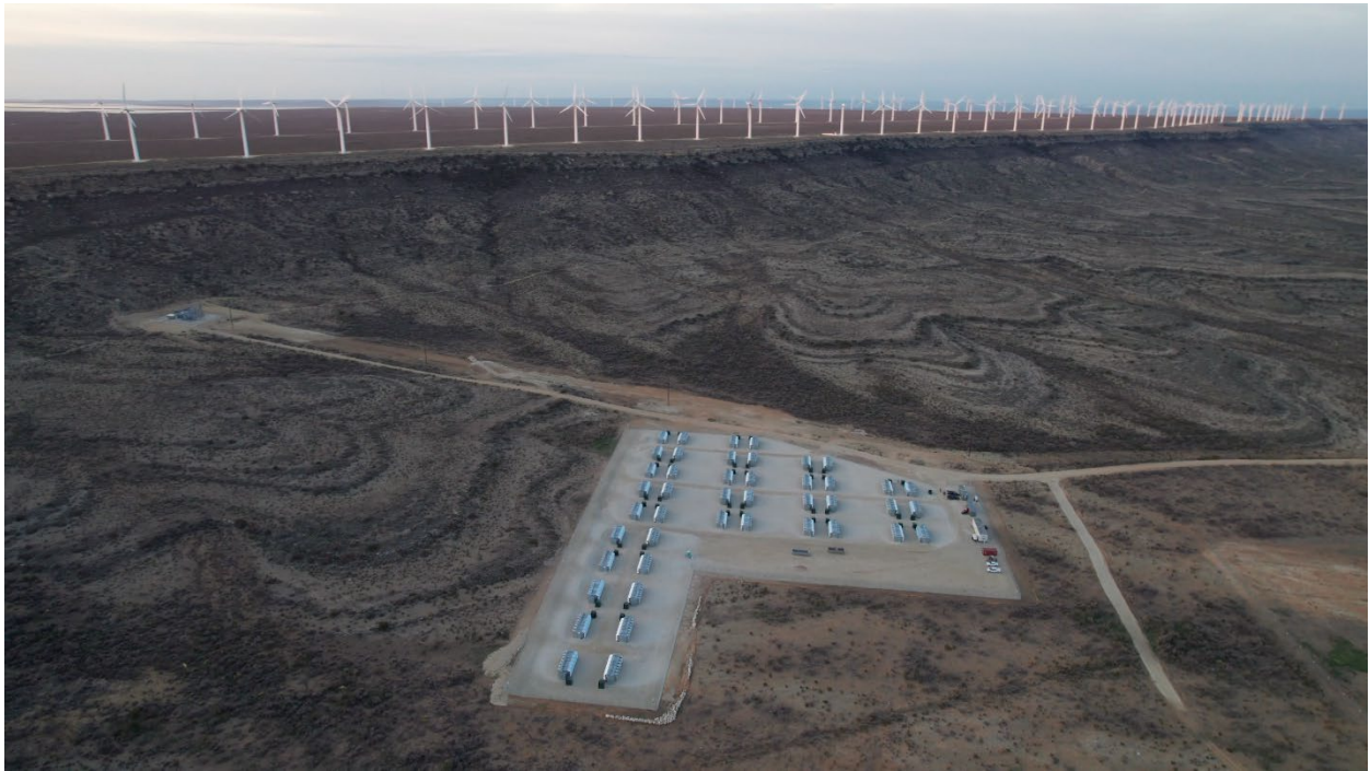
Photo of MARA's Bitcoin mining site in McCamey, Texas, where flexible load helps stabilize the grid.
