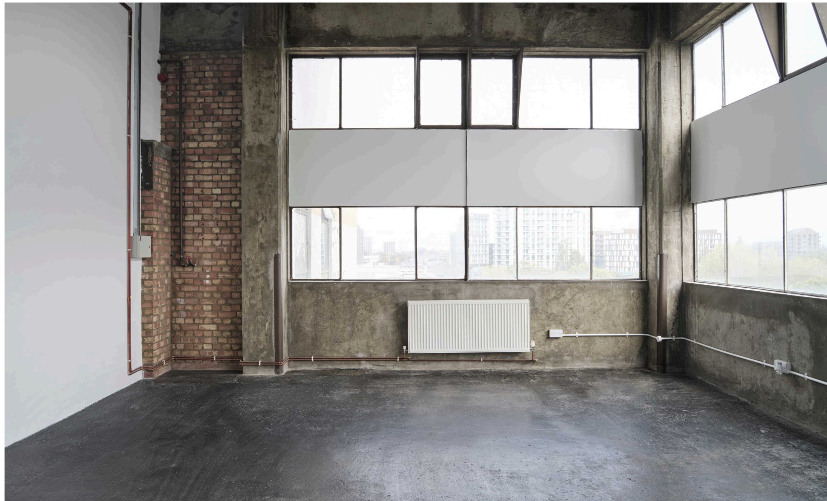
EAST AND NORTH FACING WINDOWS
