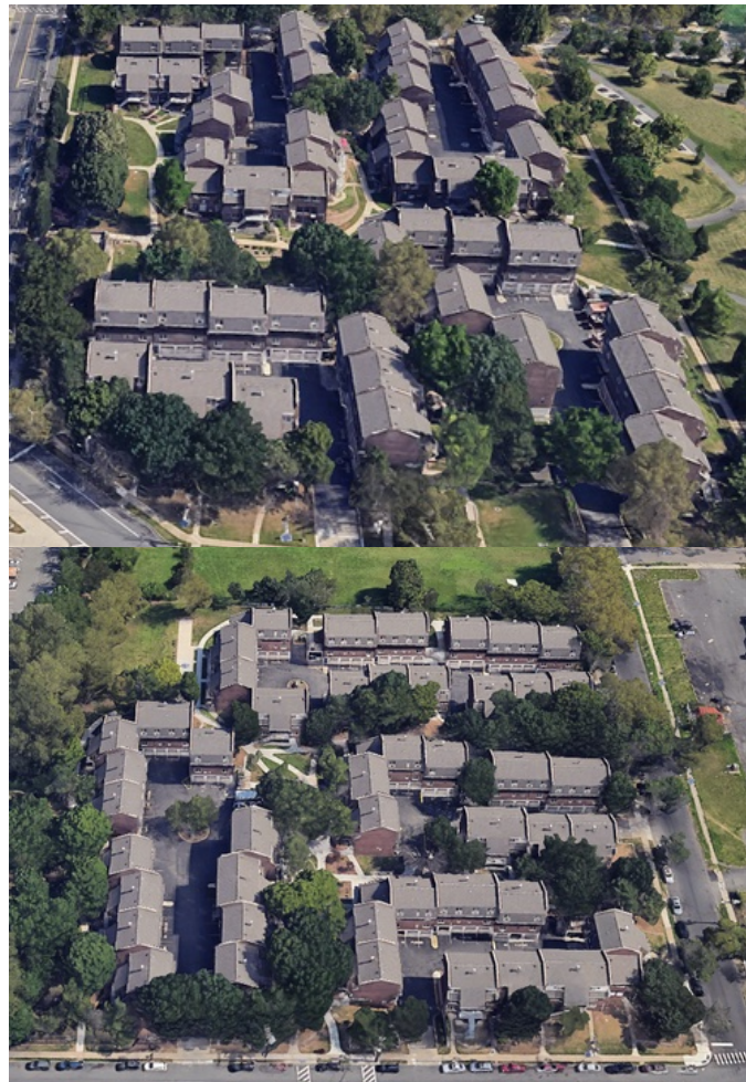
Satellite images of both garden-style properties, showing all 92 individual buildings.
