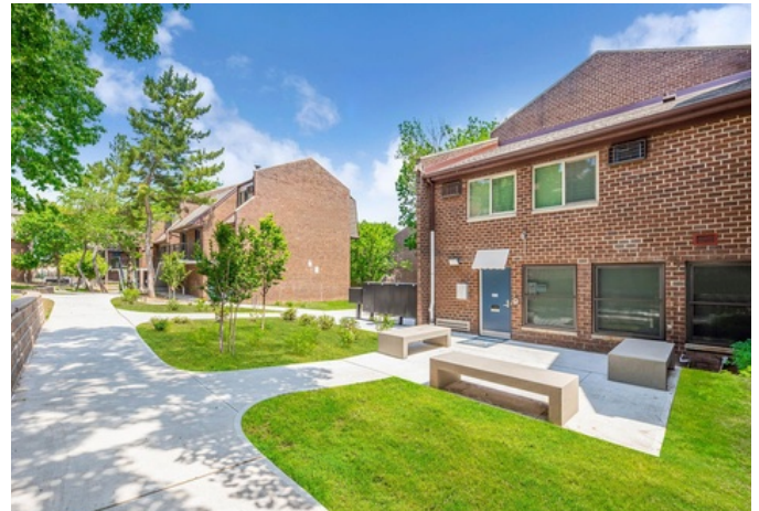
Exterior photos showing the low-rise buildings.
