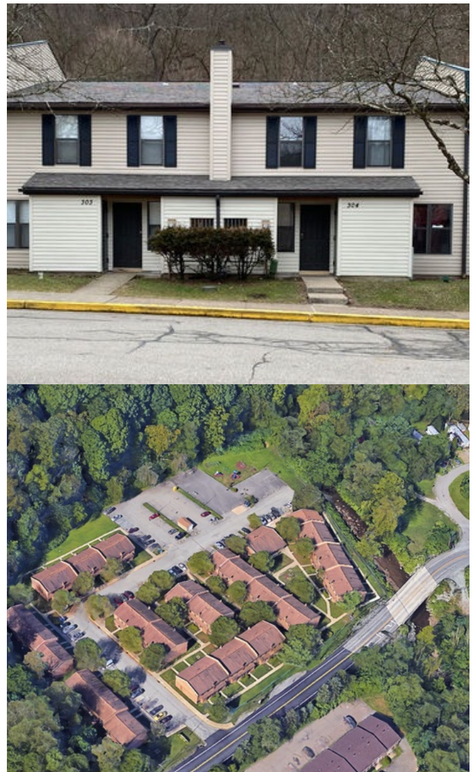
Figure 1. Above: Exterior view of a low rise building from the property in Verona, PA. Below: Satellite image of the property, showing the garden-style layout.
