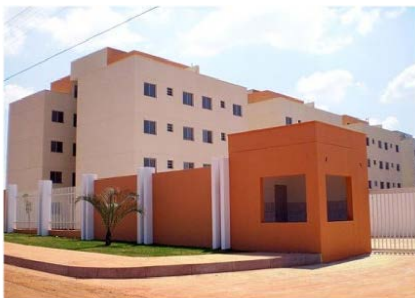
Figura 20: Residencial Multifamiliar, MCMV.
