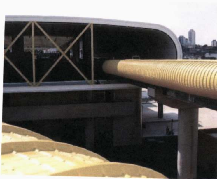
Figura 26: Expresso Tiradentes (SP) – Telha Multidobra (Fonte ABCEM, 2009)
