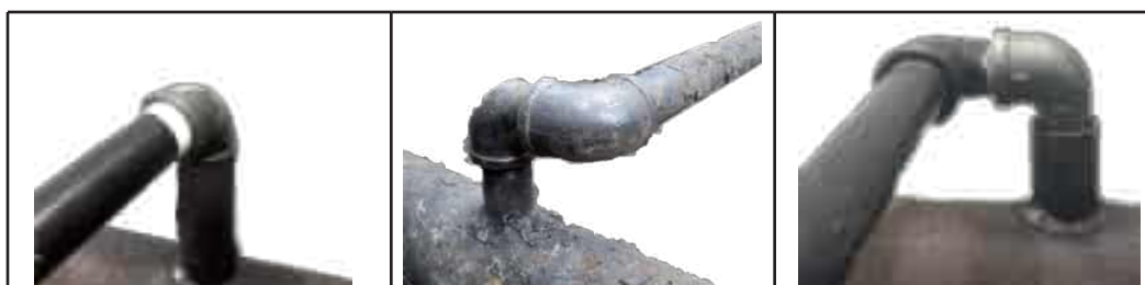
1. Elbow on TOE Nipple
