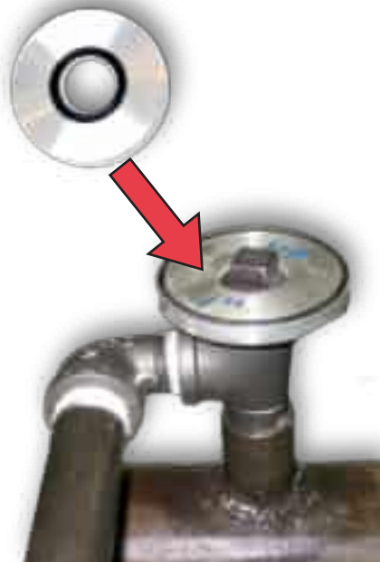
1. Disc with O-ring Seals, Around the Plug
