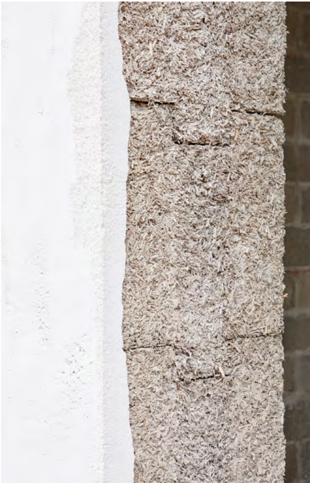
Figure 7. Interlocking hemp-lime blocks. (Image from, Parsons Healthy Materials Lab, "Designing with Hemp and Lime. Open-Source Detailing for Architects and Designers," 38-41.)
