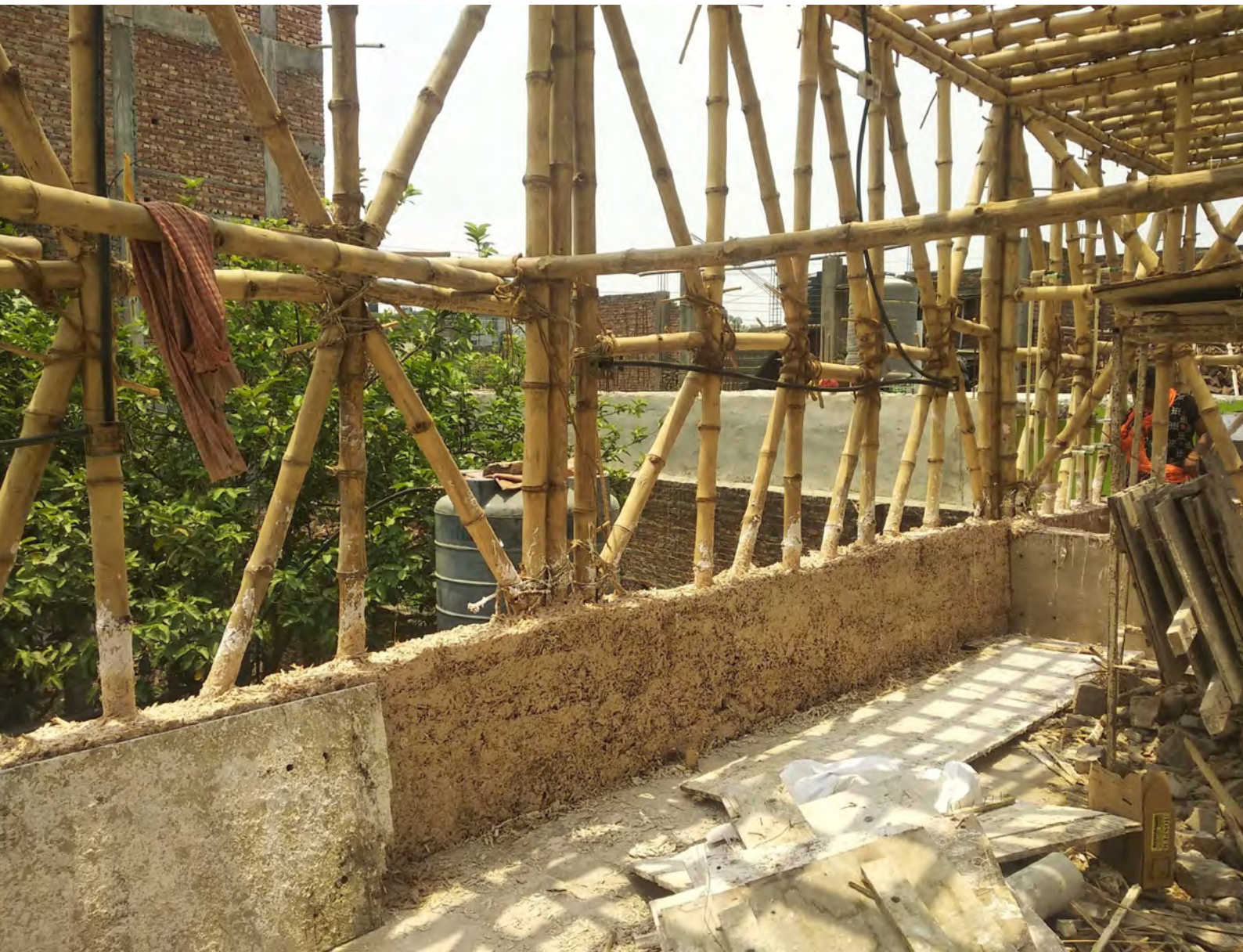
Figure 6. In-situ hemp-lime, bamboo structure. (Image from Shah Hemp Inno-Ventures, "Hempcrete Construction.")
