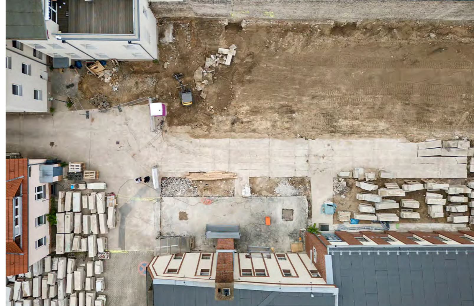
Re-use of the concrete foundation: aerial view of the B&O Bau construction site in Berlin-Weissensee, © B&O Bau; Photo: Jan Bitter, 2024
