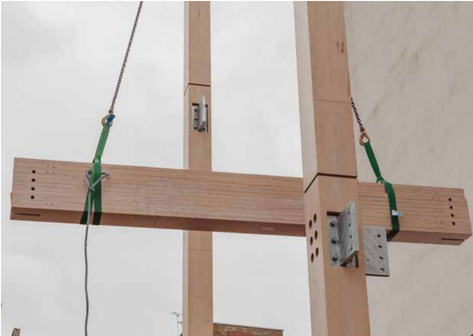
Timber structure designed for disassembly, The Black and White Building by Waugh Thistleton architects © Andy Stagg
