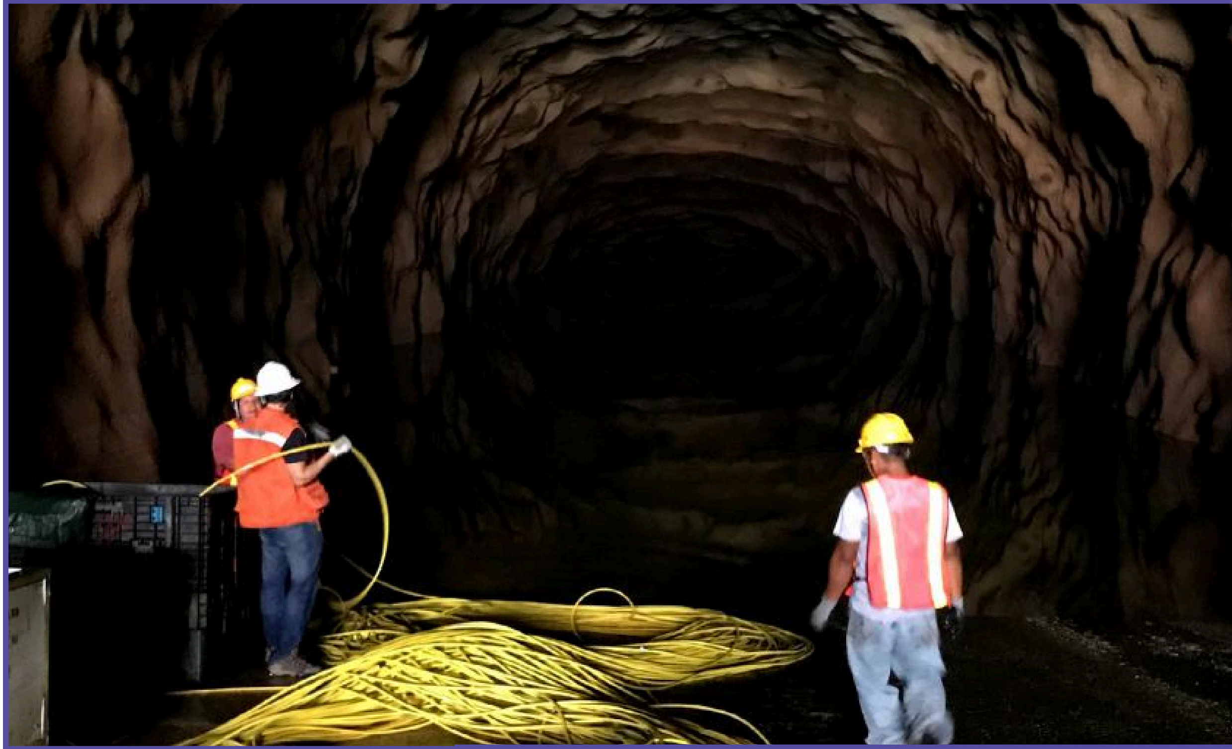
The tunnel where tests and studies were conducted
