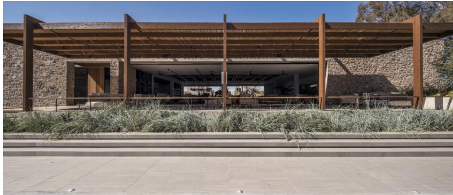
Figura 19 Fachada Principal do Hotel Theros.
