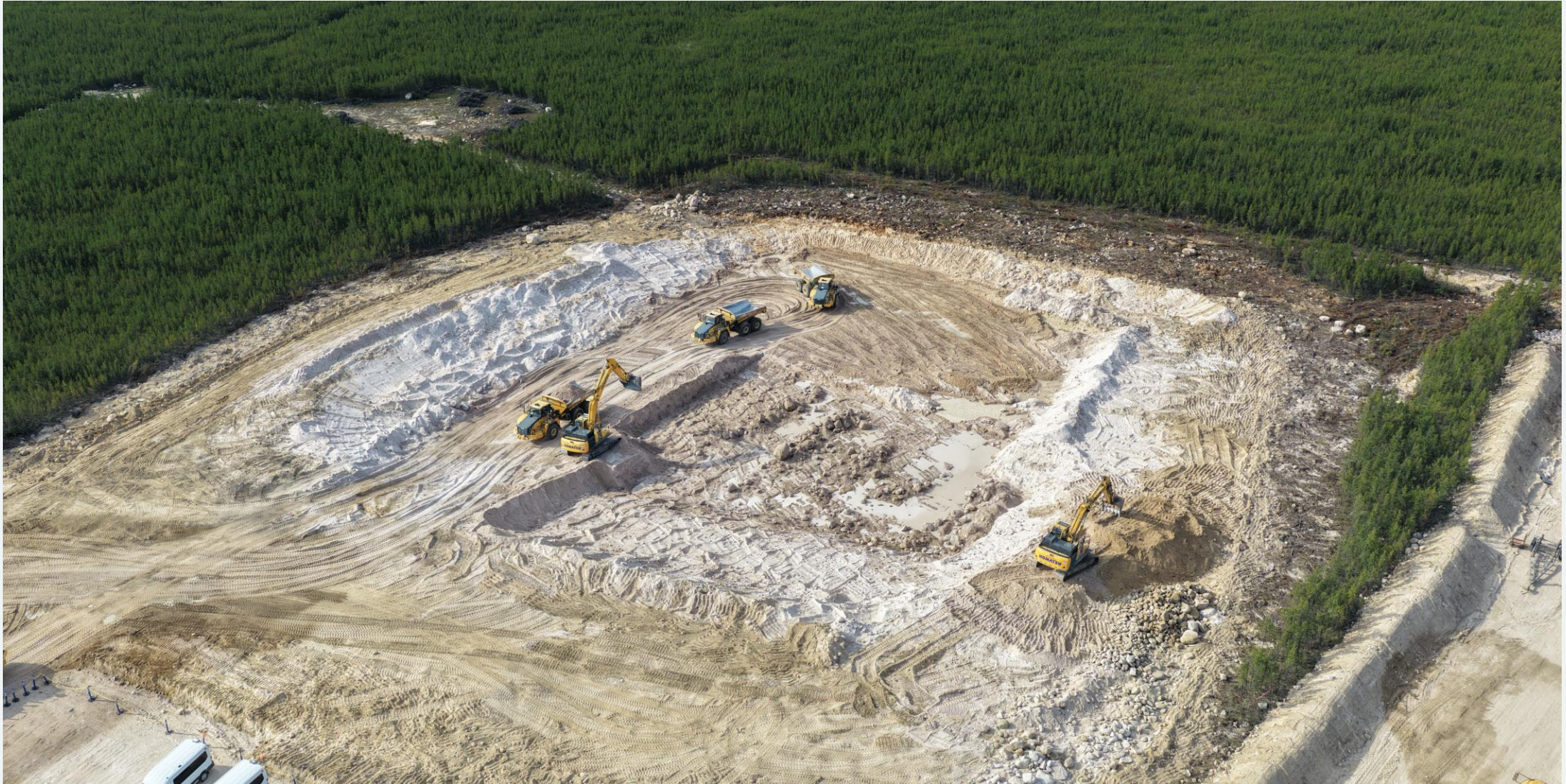
Construction facilities pad for the future batch plant and construction team offices. Stripping and grubbing completed and initial cut operation in progress.
