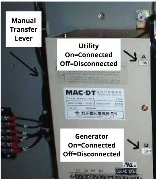
Figure 11 - Manual Transfer Lever Locations
