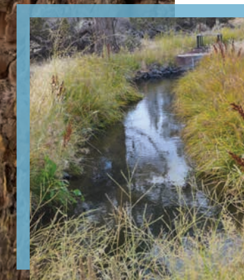
Above: Open canals lose up to half their water. Left: Lateral canals direct water from main canals.
