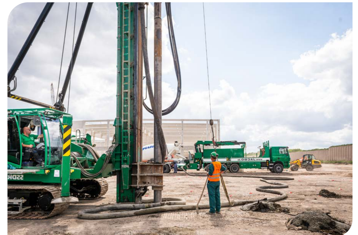
The new Woltman 130DR – digital precision and maximum reach for demanding deep foundation work
