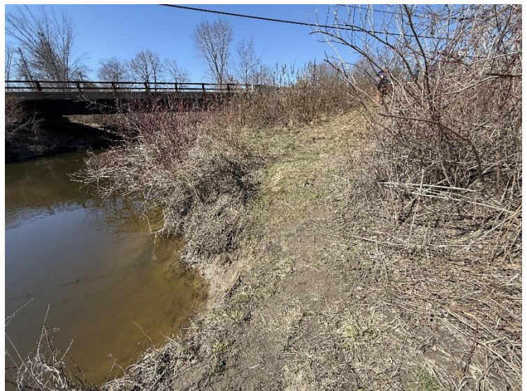
Photo 4. View of the lower launch path looking upslope.
