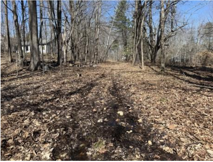
Photo 1. Wet section of trail in Segment 1. Intervale Road is located in the background of the photo.
