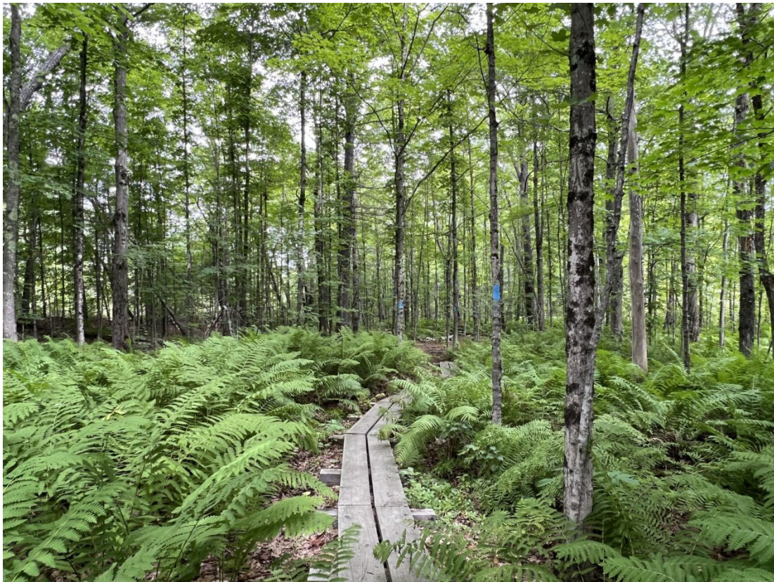
Figure 2. Existing bog bridging
