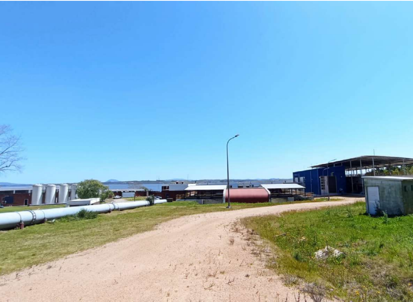
Water treatment plant located on the edge of Laguna del Sauce.
