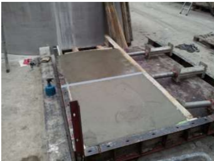
Image 1: The concrete surface after smoothing and applying of RC M040
