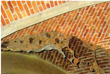
Cleaning of bricks
