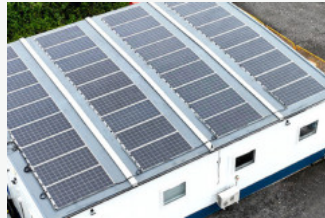
BALFOUR BEATTY MODULAR CABIN
