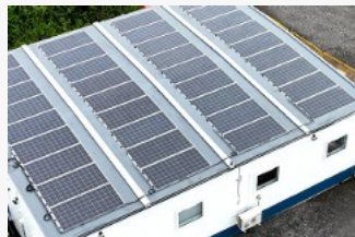
BALFOUR BEATTY MODULAR CABIN
