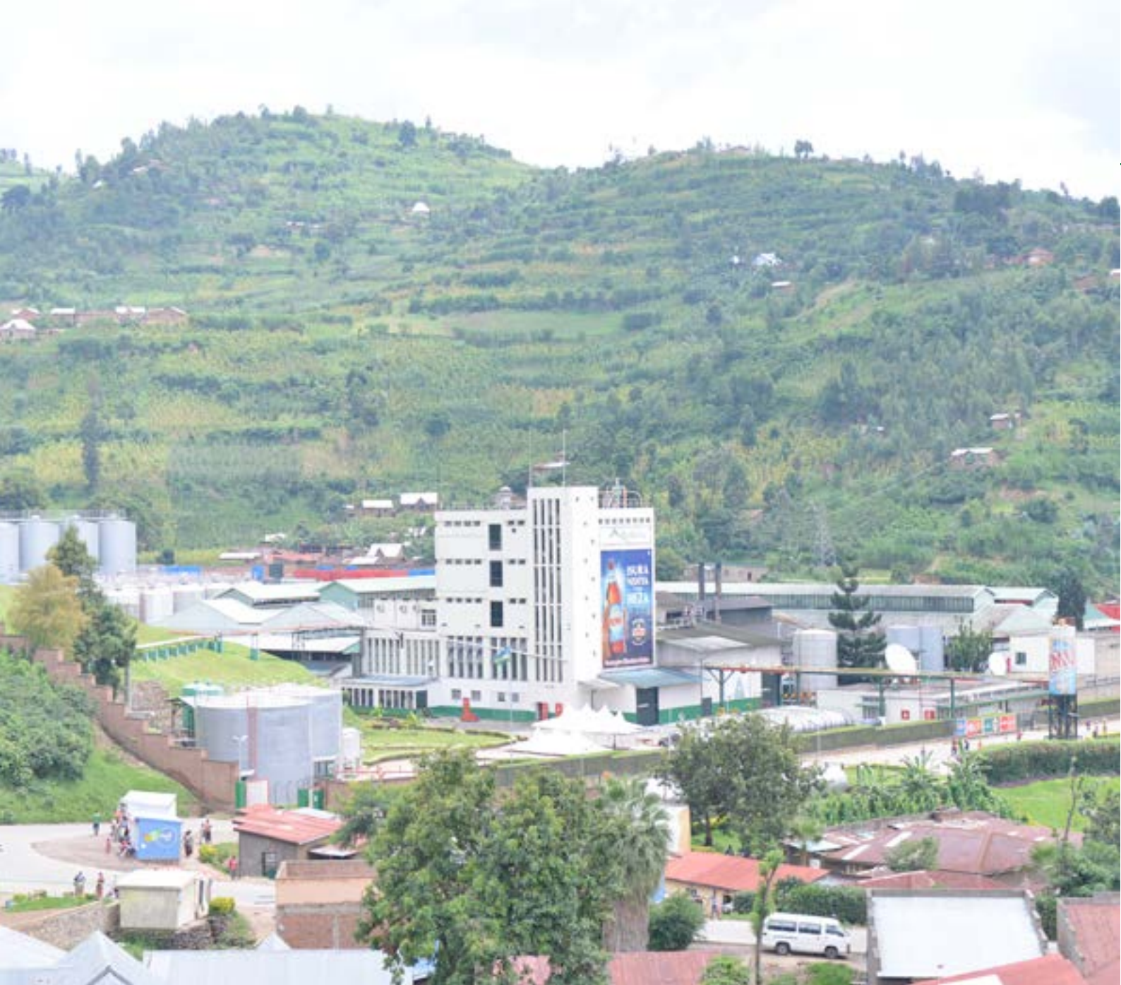
Aerial view of Gisenyi brewery site
