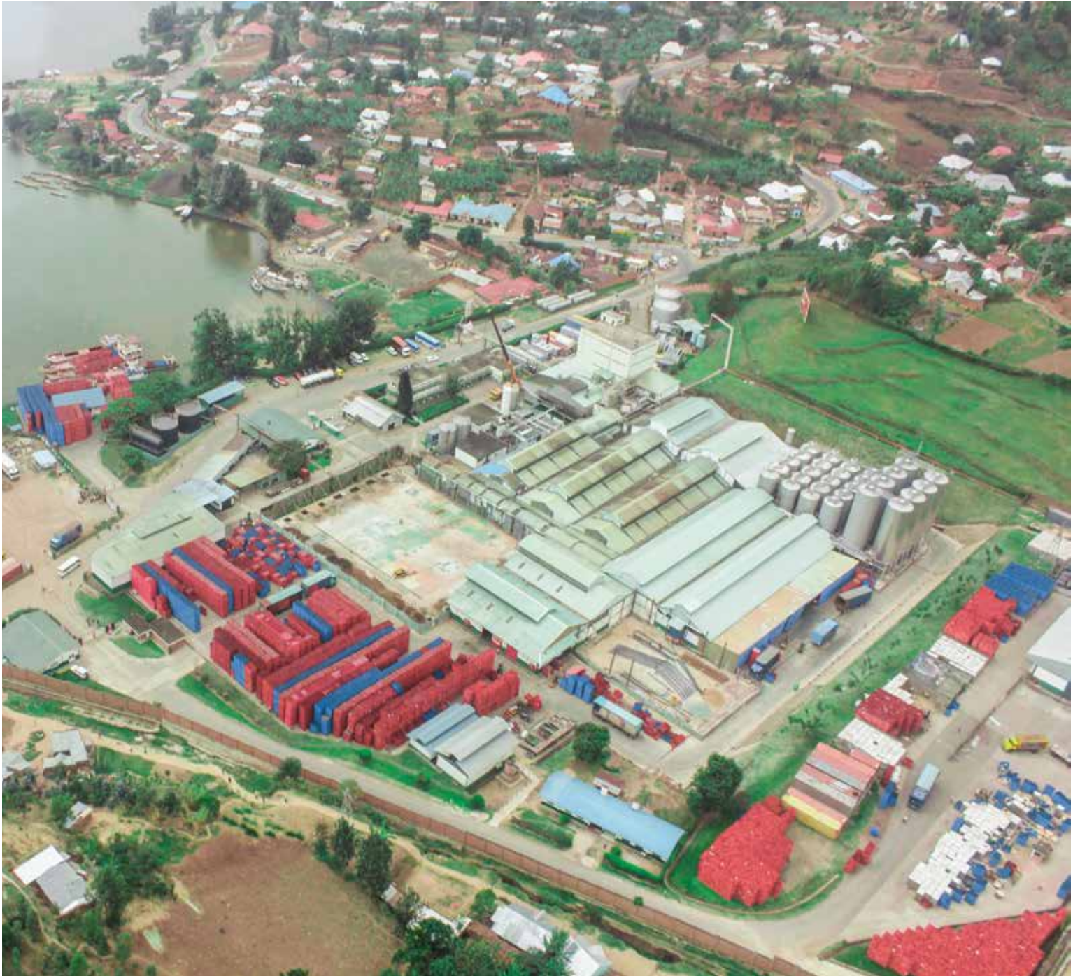
Aerial view of Gisenyi brewery site
