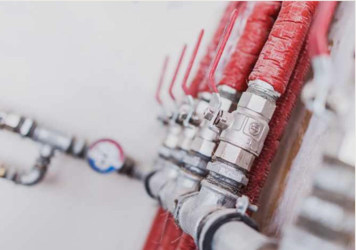
Central Heating Manifold
