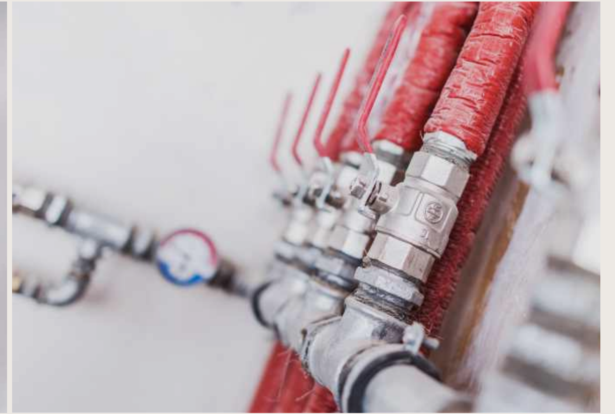
Central Heating Manifold
