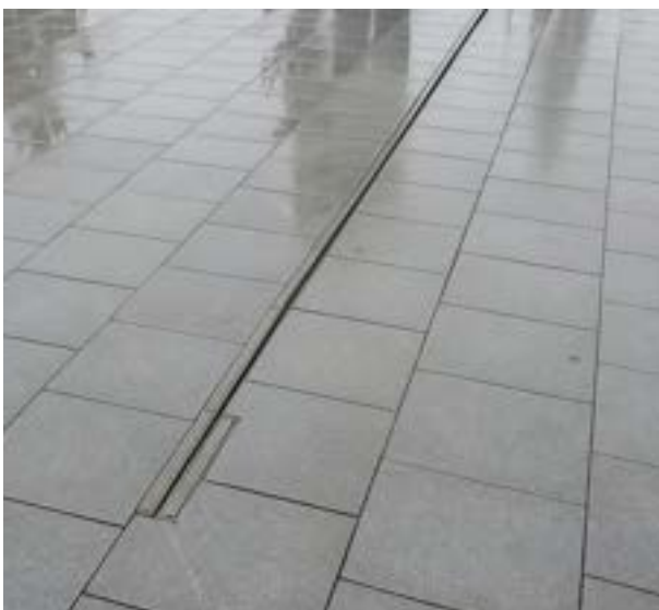
Plaza Flooring Drainage Channel
