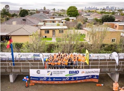
Big Bridge Build
