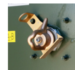
Loadbreak Switch
