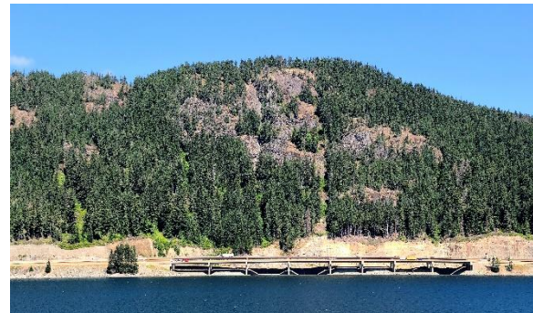
Figure 3. Snoqualmie Pass East Avalanche Bridges
