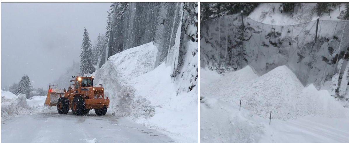
Figure 4: Attenuator rockfall nets installed primarily to reduce rockfall hazard to the highway. Avalanches both flow through the nets and are directed downward to the catchment, and to date have not adversely affected the performance of the nets.
