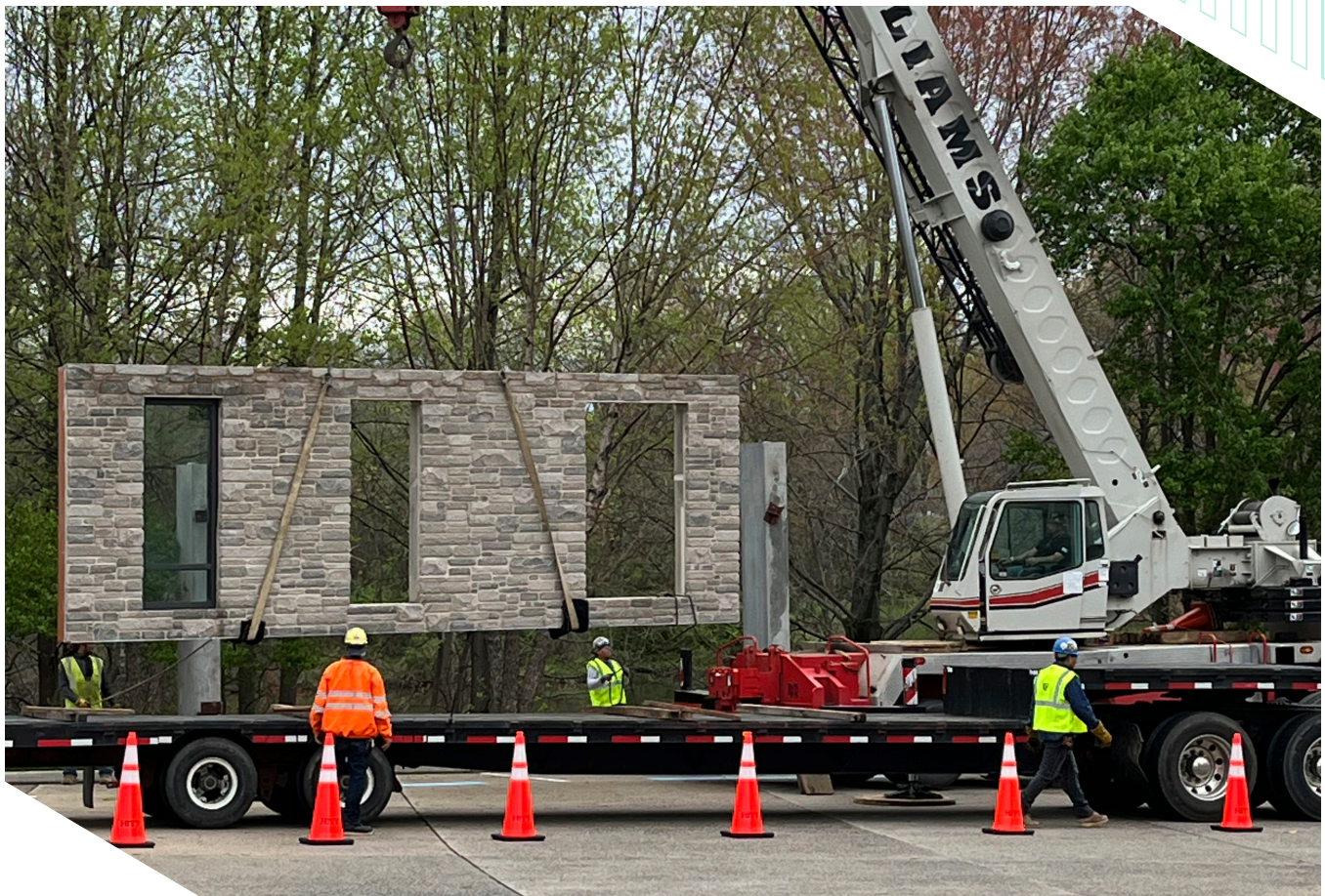
Lighter-weight panels can be moved with less-expensive equipment.
