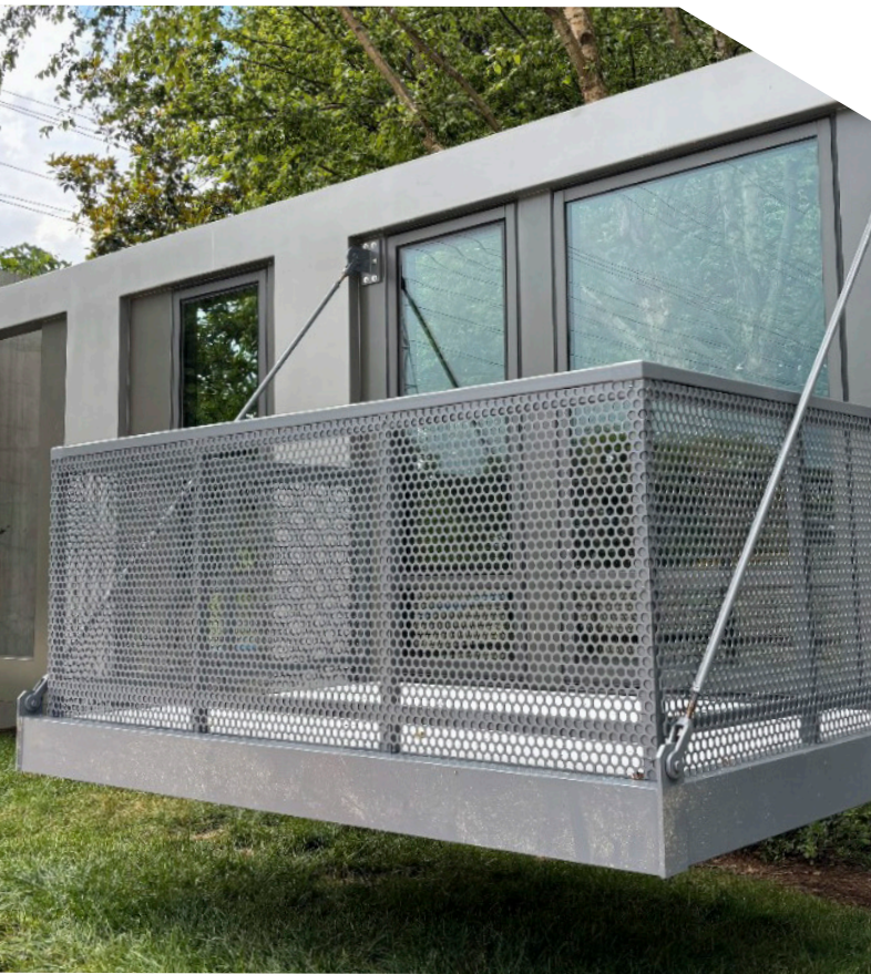
Pre-installed glazing and other integrated features reduce the number of trades needed on-site.
