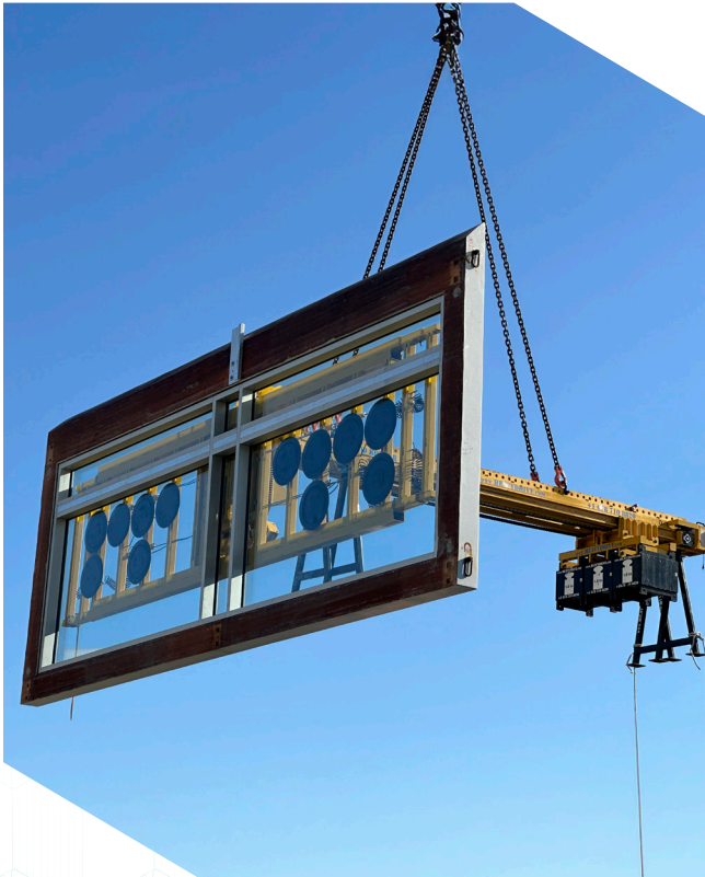
HyperWall panels with pre-installed glazing can be moved easily with a vacuum lifter.
