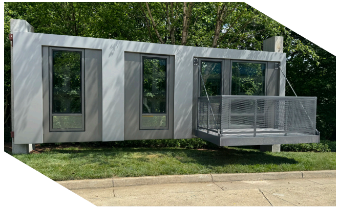
The high strength-to-weight ratio of this structural composite panel allows a balcony unit to be suspended from the panel itself.
