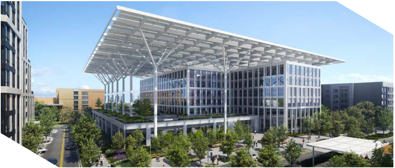
The HITT Contracting headquarters in Falls Church, Va., will feature 344 HyperWall assemblies, complete with factory-installed jumbo glazing.
