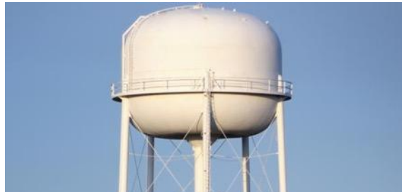
Water Tanks & Wells
